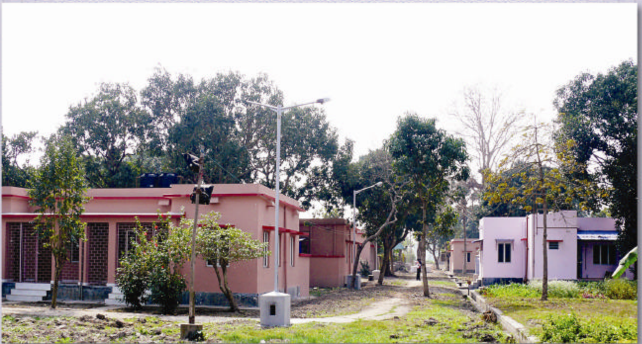
IISER-K Residential Quarters - A Partial View
